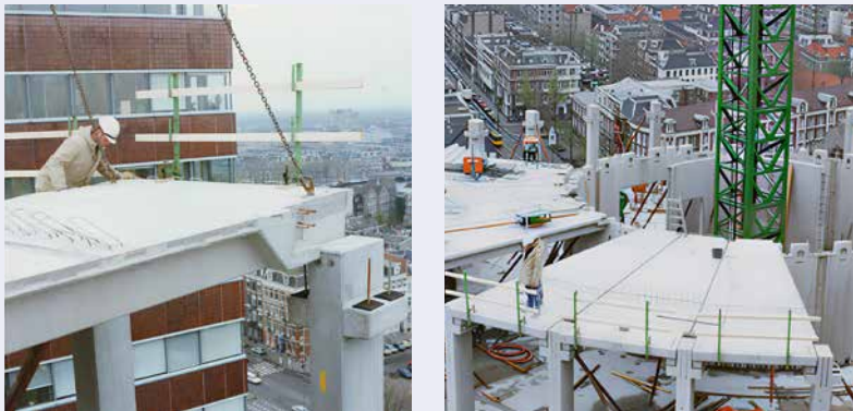
Fig. 38. De Satelliet, purchased to be demolished. ©RE:BORN
