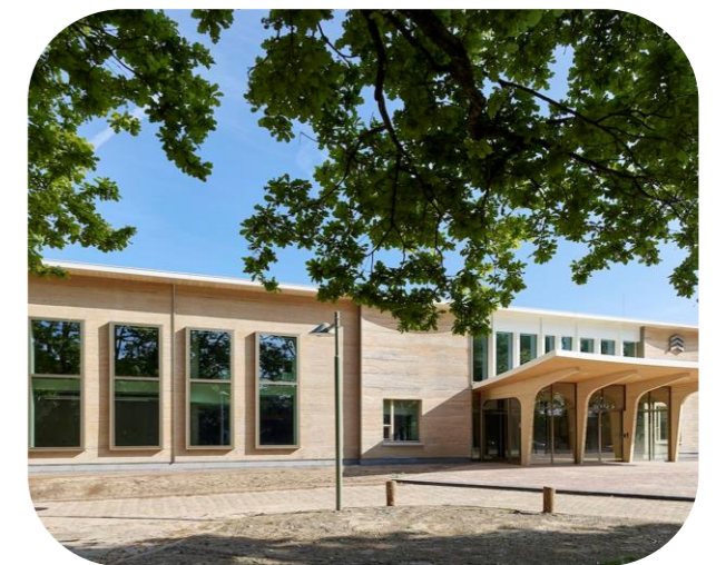
Townhall of Voorst (Hempcrete building)
