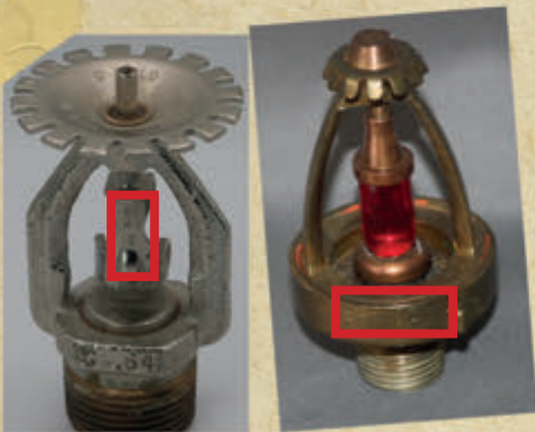
Figure 6: Date on the thermal link in small letters '98'. 1998 Reliable
